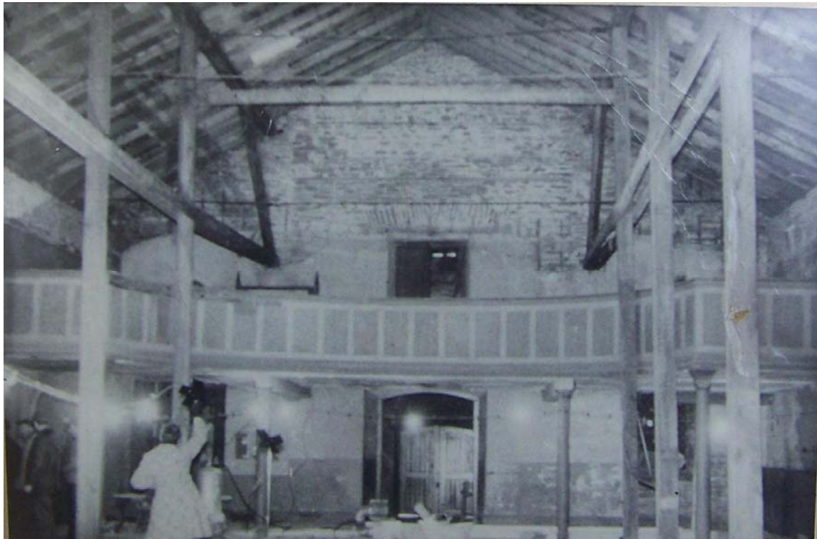
1971 Photo of Nave showing balcony detail
