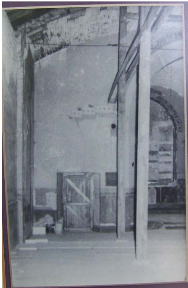
↓ East Nave Wall Showing Detail, Chancel Window and Door 1971
